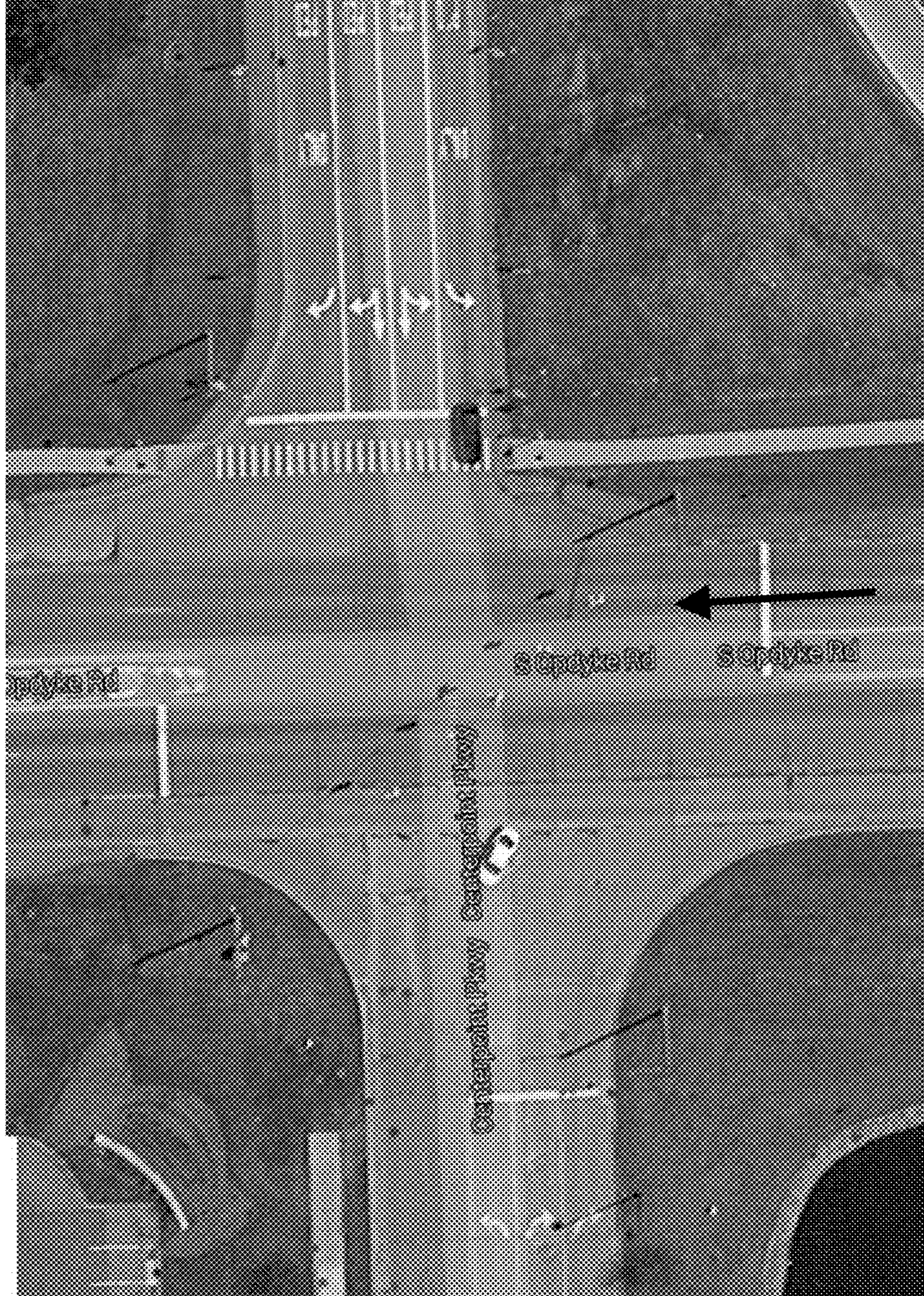
Test Results Opdyke Road / Centerpoint Pkwy FIG. 26
